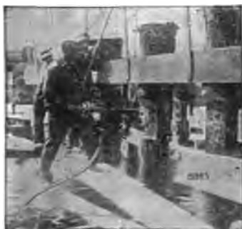
FIG. 57.—Wood-boring Machine Operated by Compressed Air.
